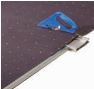
Cutting on the floor with USF. Squaring guide and hand cutter are also pictured.
