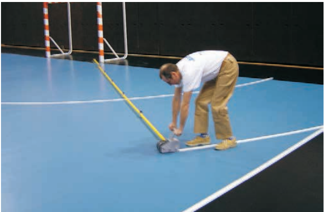
Marking Head with 50 mm marking tape
