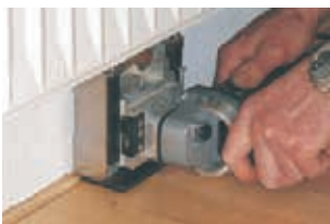
cutting expansion joints
